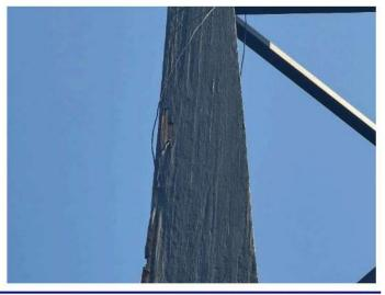
7. Delaminated paint and localized wood decay is apparent on the top of the cross member as well as immediately below the cross at the top of the steeple. Note that sheet metal caps have been installed at the tops of vertical glue-laminated members. This flashing appears to have minimized deterioration of the protected members.
