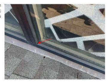
14. The protective glass was observed to have shifted at two locations, providing gaps through which storm water, as well as leaves and other debris can enter the window system (red arrows). Also note that protective glass window sealant around the perimeter of the windows is generally in a deteriorated condition and is missing at isolated locations (blue arrow).
