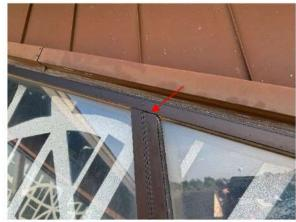
17. Sheetmetal rise-wall flashings are installed below the protective glass frame. It could not be determined whether any leaks could be related to deficiencies in the flashing without excavations; therefore, this remains a possible contributing source of water infiltration to the building interior.
