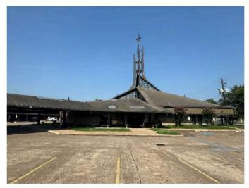
2. Photograph of the east side of the sanctuary steeple. The attachment of the four arched columns of the steeple assembly to the roof structure could not be determined. Note areas with delaminated/missing paint. Also note that wood decay is apparent within localized areas of the arched column members.
