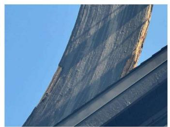
In general, the arched steeple columns exhibit uneven surfaces, which have been coated with paint. Most of the more significant deterioration is evident at the corners of the members.
