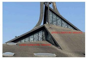
frames with perimeter sealant. Protective glass is provided on the outside of the original window frames using aluminum frames and perimeter gaskets.
