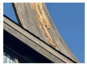
View of the base of the south arched column member of the steeple. Rotten wood is apparent at the corners of the member; however, the interior wood generally appears to be in acceptable condition.
