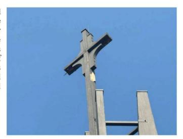
8. Steel framing members tie vertical members of the steeple together (photograph provided by St. Andrews). The steel members and bolted connections appear to be in good condition. It should be noted; however, that the base of the center vertical member of the cross exhibits deterioration. The extent and severity of the deterioration was not apparent from the vantage point of the Close-up inspection photographer. will be required to determine appropriate corrective action.
