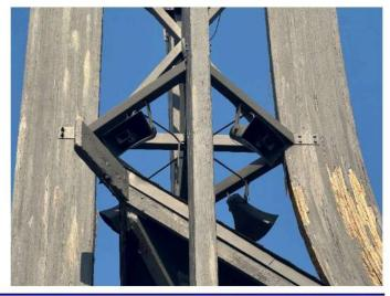
Close-up view of water-related deterioration at the base of the north arched steeple column. Similar distress is also apparent on the other three other columns, particularly the one on the west side.
