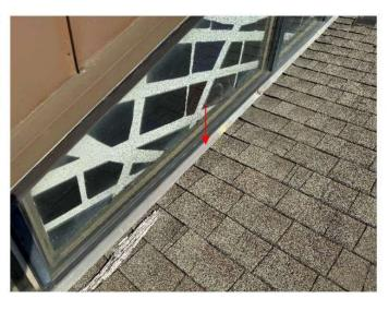
18. Flashing is provided at the transitions between the various roof levels and sealant is utilized to seal the flashing to the substrate. The sealants are typically in a deteriorated condition due to normal aging. In addition, deterioration of the wood rakes is apparent at the flashing locations.
