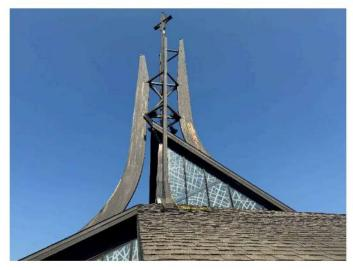
3. Close-up view of the arched steeple columns. Note the missing paint and apparent minor decay of the underlying glue-laminated member.
