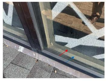
13. Gaskets for the protective glass were observed to be in fair condition; however, shrinkage has resulted in gaps forming at the window corners.
