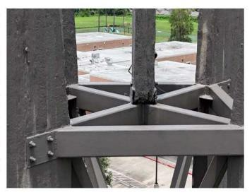
9. The ridge beam extending out from the southeast corner of the upper roof and the rake/fascia that frames into the ridge beam exhibit severe deterioration. The photograph below on the left was documented from the southwest and the one on the right was documented from the east, looking upward.
