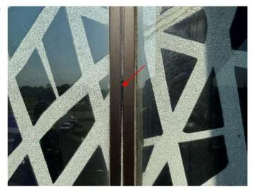
16. Sealant has been remedially applied over some, but not all joints in the protective glass aluminum frames.
