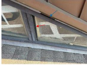
15. Sealant was applied to the joints of some lower clerestory windows; however, the sealant is exhibiting deterioration due to normal aging and is missing at isolated areas. Typically, no sealant is provided in these joints on the upper clerestory windows.
